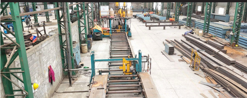
PULL THROUGH WELDING
